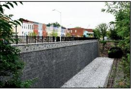
**Project Description and Specific Nature of Work:** As the constructor, CGI was responsible for all construction including roadway, retaining walls both temporary and permanent, sidewalks, street lighting, signing, pavement markings, utility coordination, E&SC, and public outreach. **CGI also coordinated and partnered with the Project Designer, WRA.**
